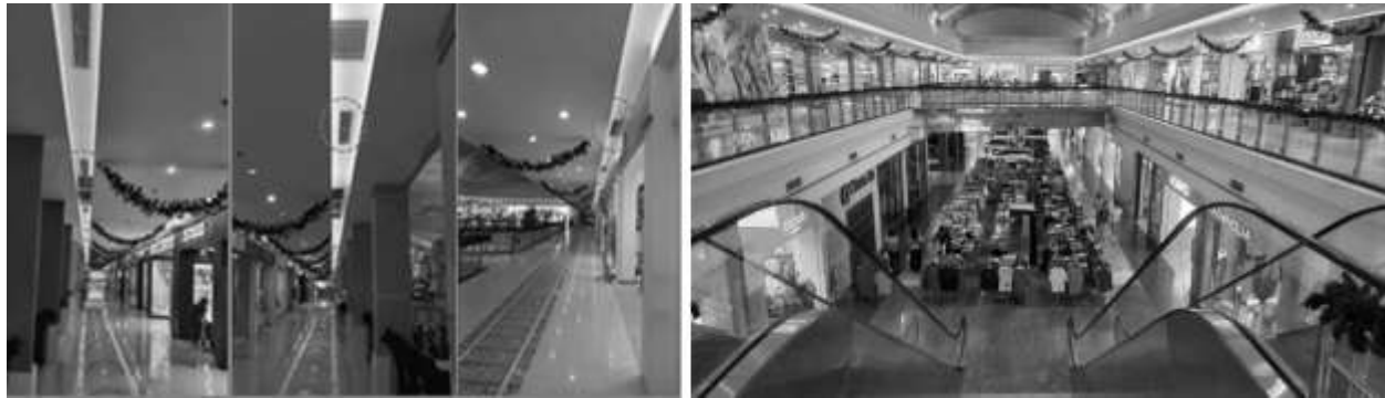
Figure 2. Air-supply diffuser installation in the atrium and corridor areas
